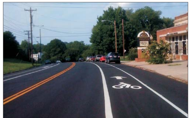
The repaving of Northwest Boulevard included parking and bicycle lanes from Hawthorne Road to Reynolda Road.
