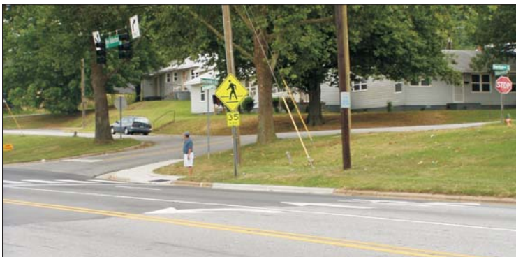
New Walkertown Rd at Overlook Dr before ARRA project improvements.
