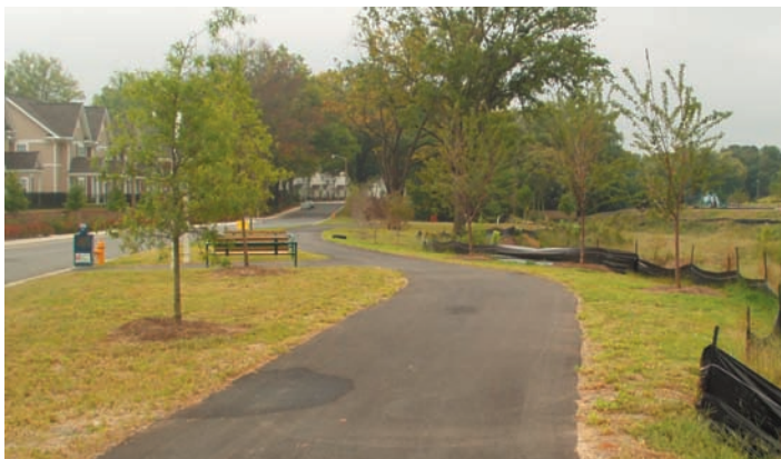
A shared-use path at Drayton Pines Park.
