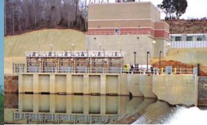
Northwest Water Treatment Plant's dam and pump station is capable of pulling 50 million gallons a day out of the Yadkin River.
