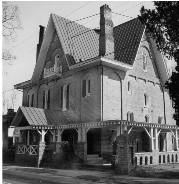
Korner's Folly, located near the center of Kernersville is one of Forsyth County's most well known nineteenth century residences. Visitors young and old marvel at the unique architecture of the building, with its many rooms, twenty fire places, alcoves and passageways. The building is on the National Register of Historic Places and is a local historic landmark.
