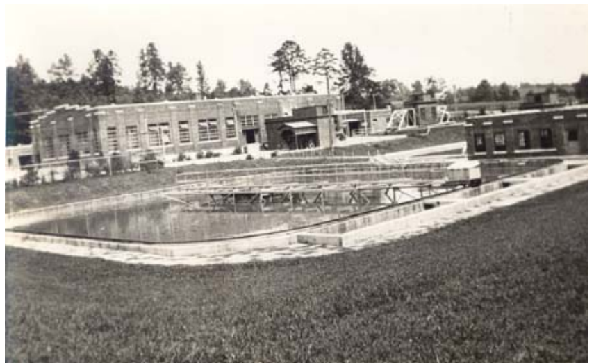
The Salem Water Plant off Stadium Drive would be renamed for Public Works Director R.A. Thomas in 1951. (Forsyth County Public Library Photo Collection)
