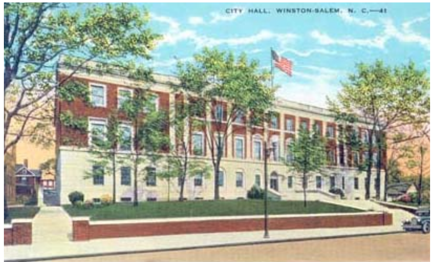
When City Hall opened it was the largest municipal building in North Carolina. (J.R. Snider postcard collection)
