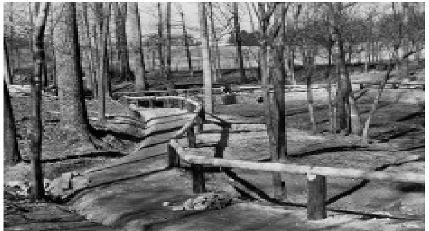
The trail in Miller Park. (Forsyth County Public Library Photo Collection)
